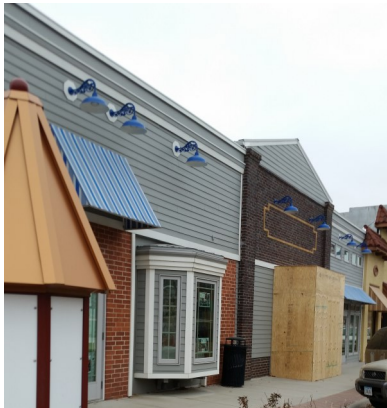
105 N. Elm is being renovated to welcome American National Insurance.
